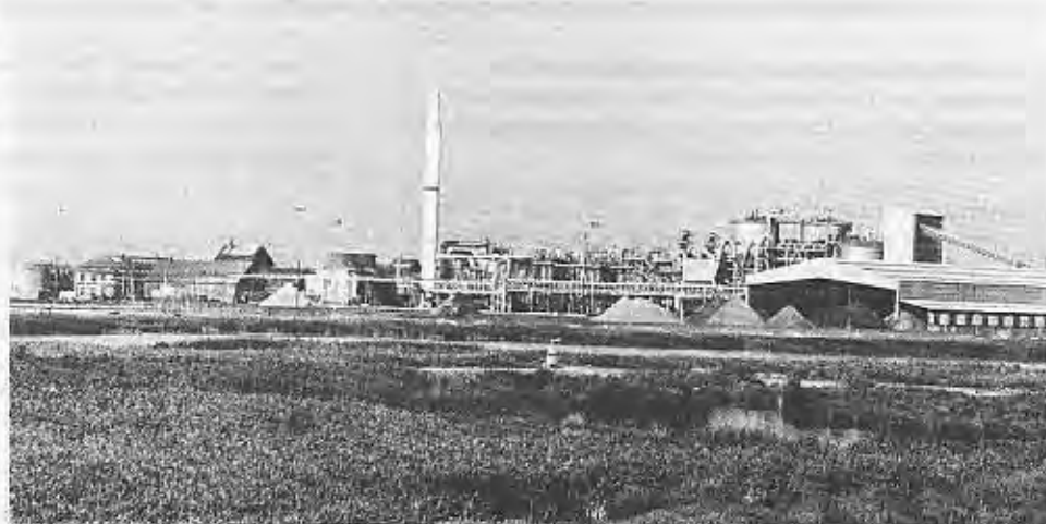
FIGURE 24.33 RTZ Electrolytic Zinc Plant at Budel, Holland
