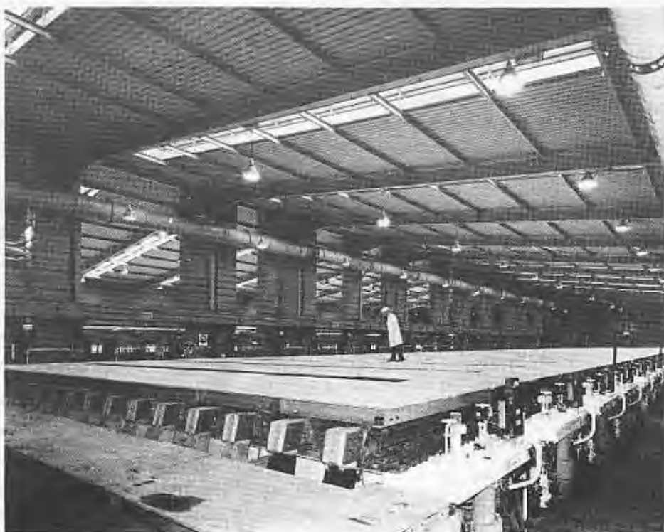
FIGURE 18.4(b) Mercury Cathode Cells at ICI, Runcorn
