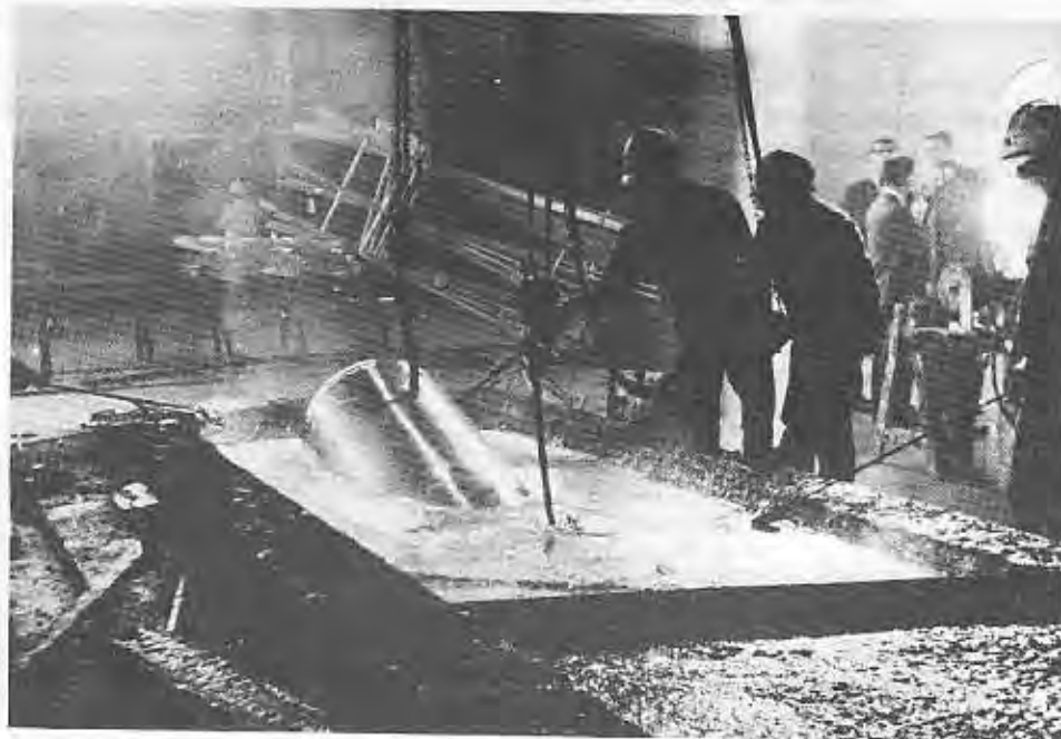
FIGURE 24.28 Galvanising a Metal Container
