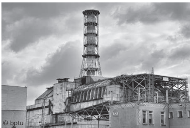
Fig. 23.10 The remains of the Chernobyl nuclear power station. The site will remain a prohibited area for many years
