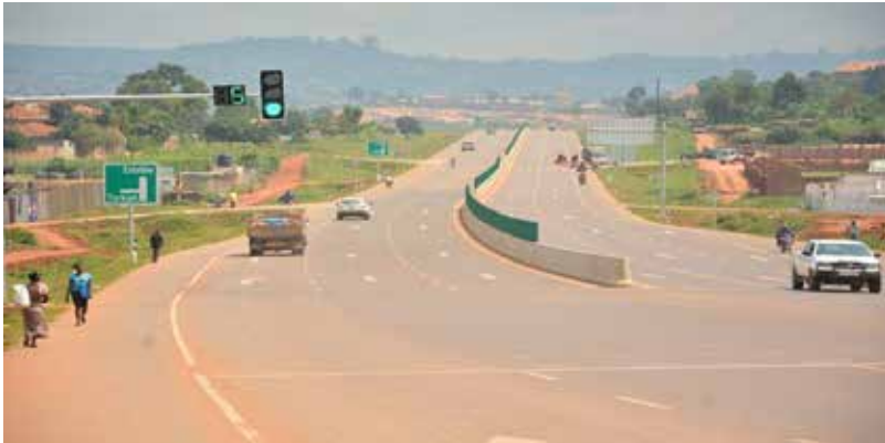
Figure 3.3: A section of Kampala- Entebbe express highway
