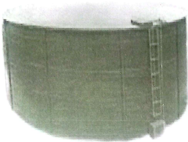
Fig 2. The cylindrical metallic water tank
