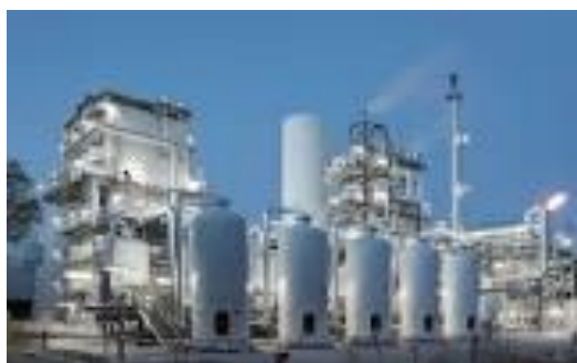
Fig. 2 An Oxygen Plant
