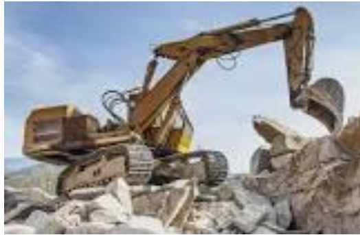
Fig 4 showing a Rock Quarry
