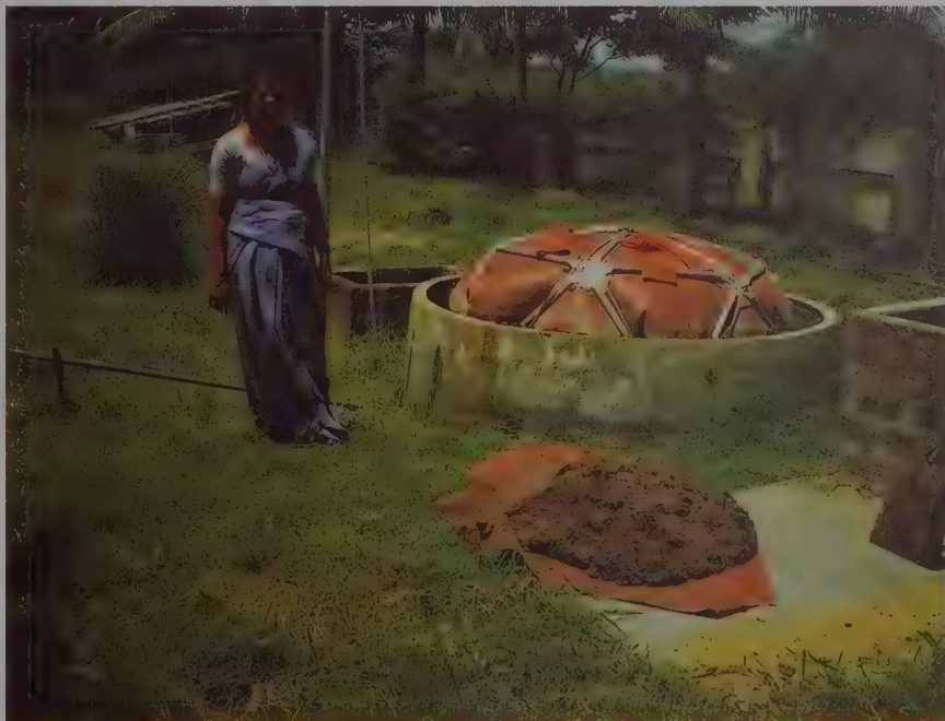
Figure 5.26 A domestic 'biogas' digester in an Indian village, using animal manure and producing methane for cooking and heating water
