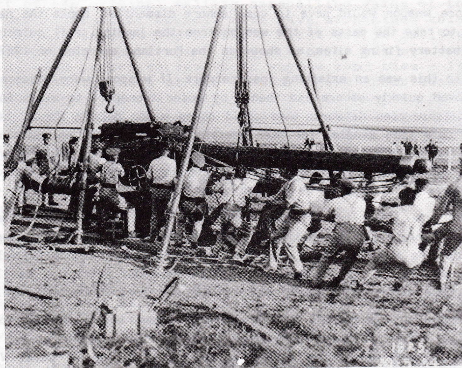
"A 6 inch gun being mounted in a cradle at Fort Cumberland 1933"
