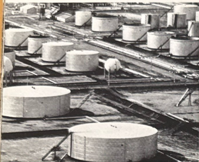
Thirteen million barrels of crude oil and products can be stored in Amuay's installations of traditional steel tanks.
