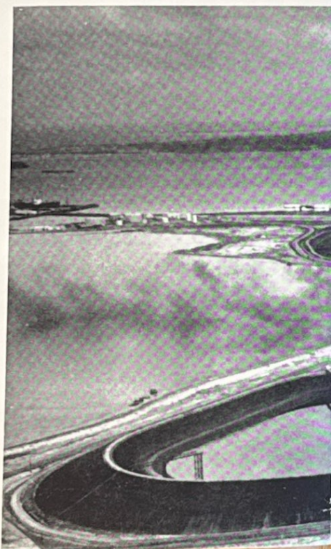
Twenty million barrels of fuel oil can be stored in the two open air tanks seen in the foreground and at the center. A smaller pit between them is used to filter sea water that has been used in refining processes.
