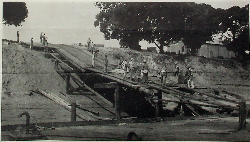
Ramp used in unloading materials from SS Bolivar at La Pena Terminal. This is one of the difficulties confronting wildcat operations of Venezuela Gulf Oil Company in Eastern Venezuela.
